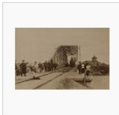
View after completion of the bridge
