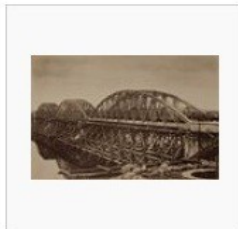
Construction of the bridge deck
